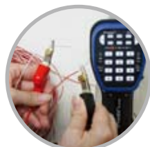
Line Continuity Test
