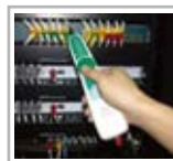
Copper cabling detecting, including shielded (STP) and UTP cable
